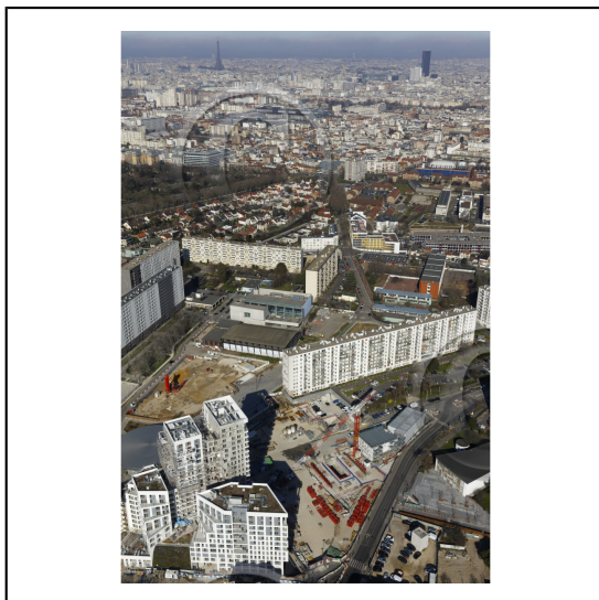
92 Hauts-de-Seine R?gion ?le-de-France / Bagneux : Travaux de construction de la gare de Bagneux du Grand Paris Express GPE ligne 15 / La gare SNCF de Bagneux / Paris en arri?re plan *** Local Caption *** Bagneux: The new railway station Bagneux under construction / The project GPE Grand Paris Express line 15/ The railway station SNCF Bagneux / 92 Hauts-de-Seine R?gion ?le-de-France
